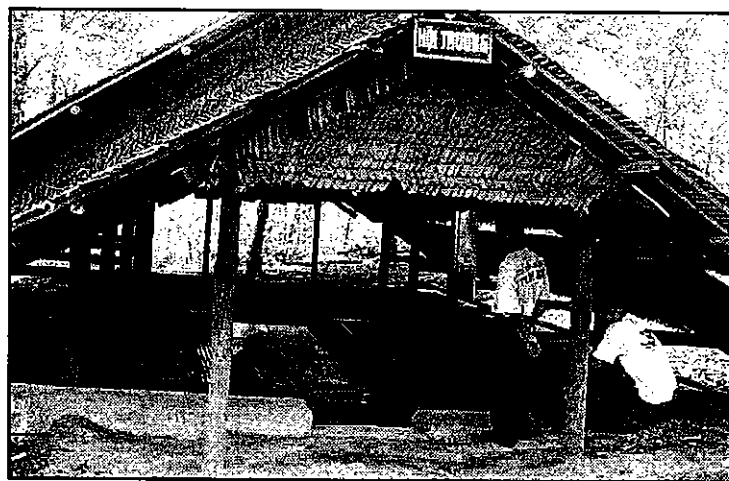
Restored shelter at COSVN Headquarters near Xa Mat, Tay Ninh area
